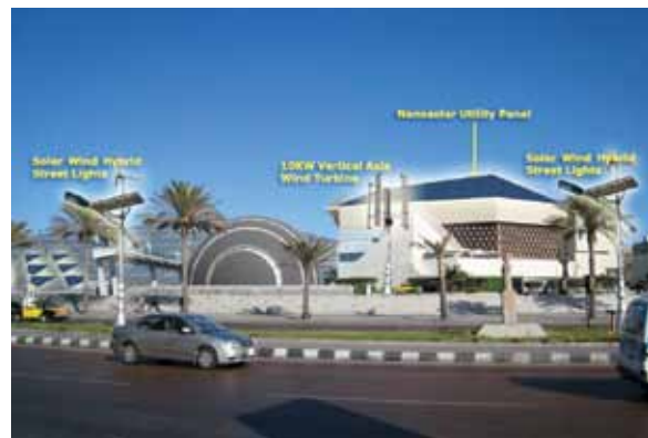
External elements of renewable energy sources on the BA Plaza
